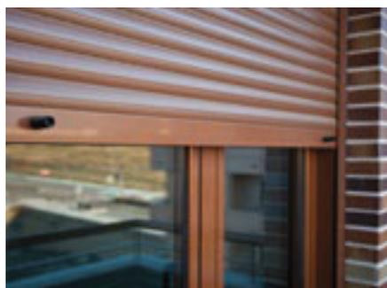
(such as louvres, overhangs and fins) are widely used in the UK, the thermal benefit of the external thermal roller blind device has not been fully realised and such devices are currently used for security purposes.
